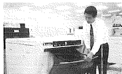
Page-Negatives/Plotters Each plant receives page images from the Tokyo headquarters, then page negatives are made by plotters. Aluminum printing plates are then made from the negative film.
